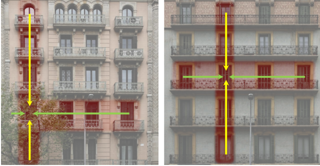
Figure 2. Facade layouts present strong regularity, as the architectural elements are well-aligned both vertically and horizontally. The spatial correlation between facade elements in the two directions provides valuable context for facade element detection.
